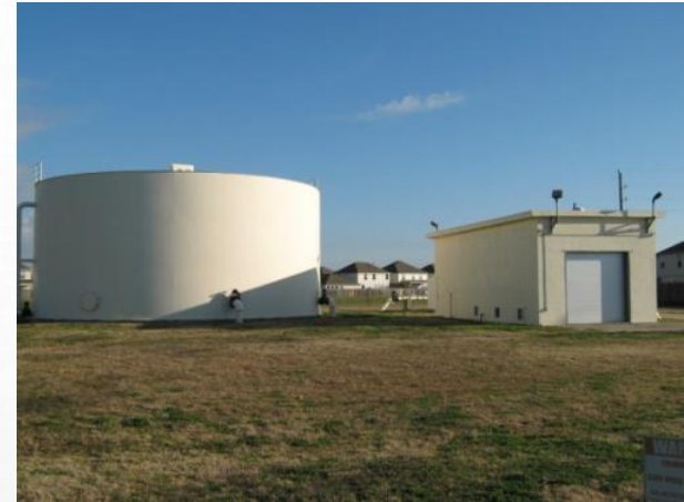
Water Plant No. 2 in Lake Ridge Subdivision
